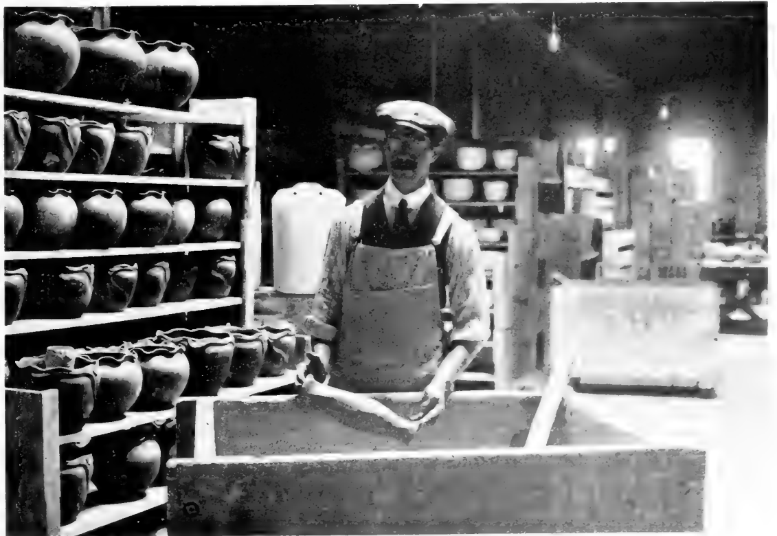
Dipping into the Glaze after First Firing
